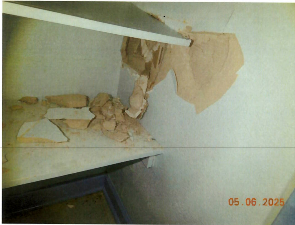
Photo No. 11: Puncture in the wall between the hallway closet and bedroom 2.
