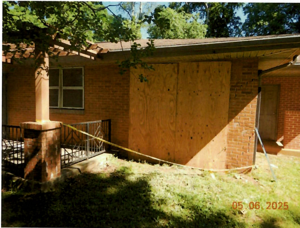
Photo No. 4: Boarded over double window in the south wall of bedroom 2.
