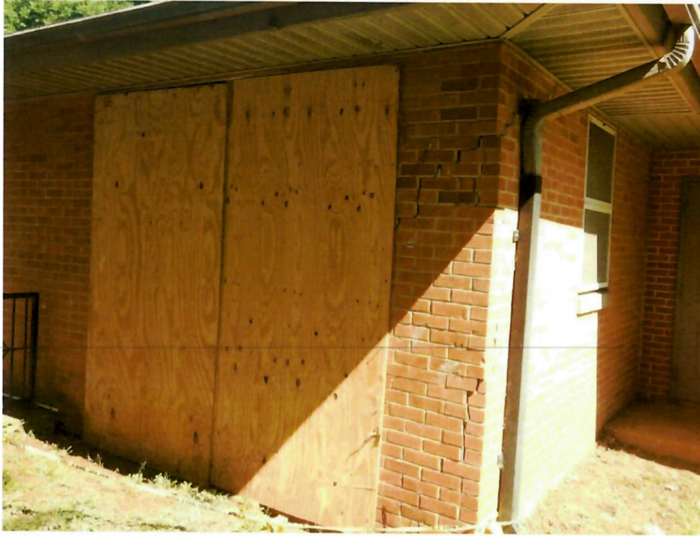
Photo No. 5: Cracked and displaced brick veneer at the southeast corner of bedroom 2.
