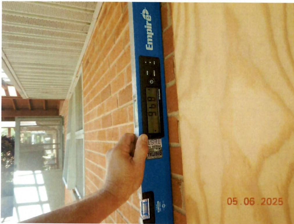
Photo No. 6: Outside the damaged area the brick veneer was plumb.
