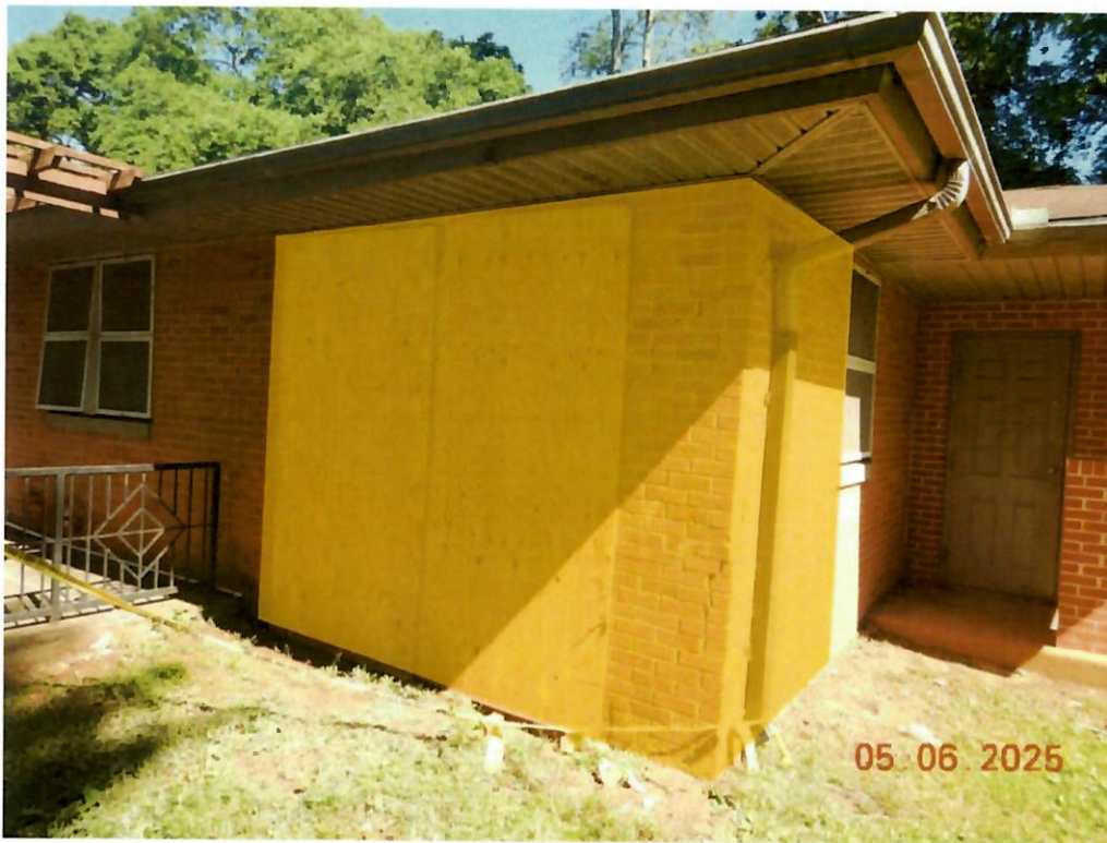
Photo No. 14: Damaged area of brick veneer that should be removed.
